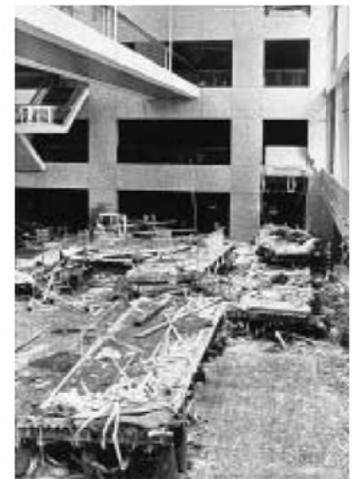
**FIGURE 12-1** Elevated walkway collapse in a Kansas City hotel in 1981. How a simple physics calculation could have prevented the tragic loss of over 100 lives is
