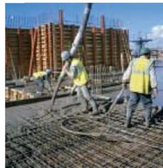
**FIGURE 12–22** Steel rods around which concrete is poured for strength.
